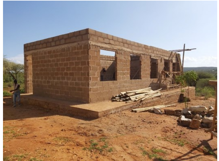
Laborbau an der Mandaka Secondary School
