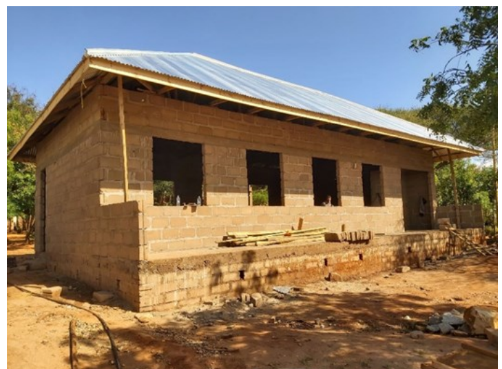
Laborbau an der Vudoi Secondary School
